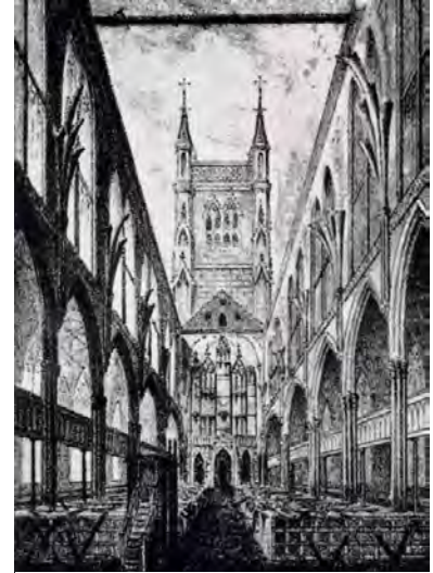
The Nave after the fire
